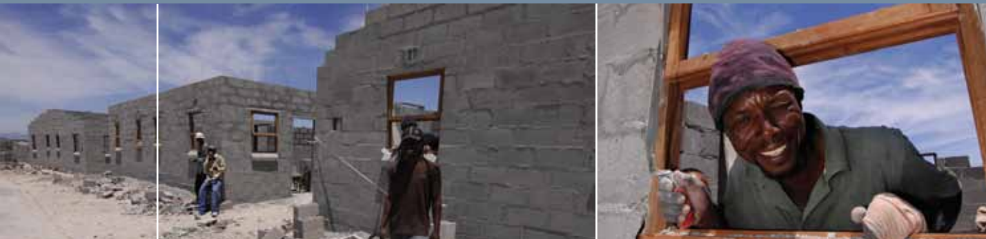
New housing projects involving local labour
