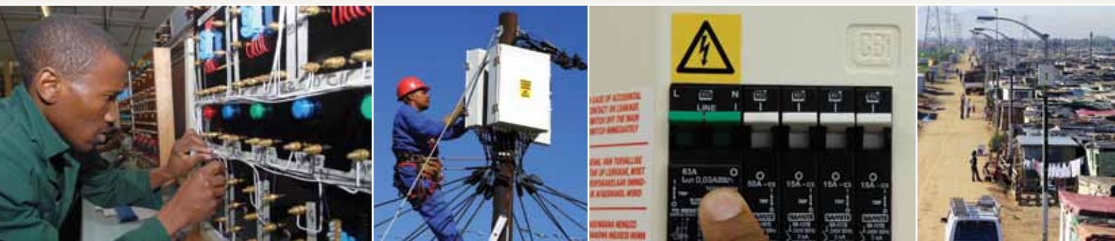
The City provides electricity distribution services to approximately 75% of City customers
