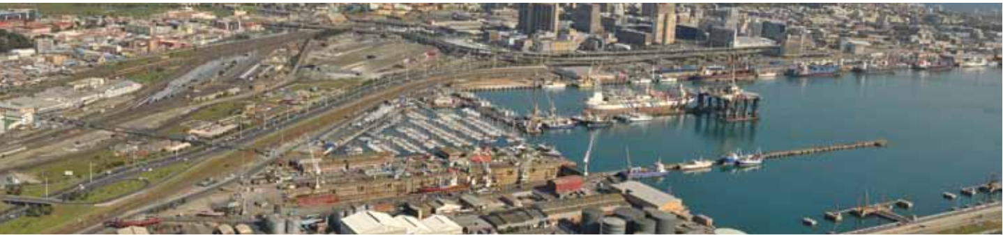
Cape Town Port is set to undergo a major expansion
